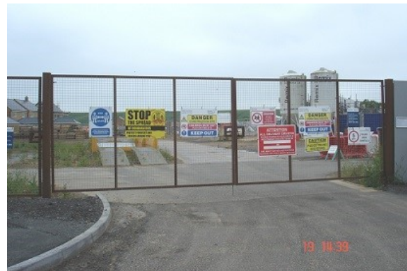
295 Bovis Homes under construction in 2022
