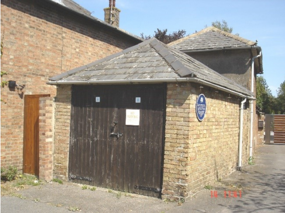
Fire Pump Accommodation
